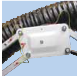
Joint Intermediate plates at top joint with relief cables between construction parts.
